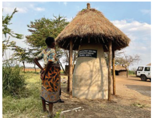
Figure 3. A woman stands in front of an elephant-proof grain store installed by FZS in Tanzania; cement/brick stores like this are used to protect grains from elephants. (© Lucy King/Save the Elephants)
