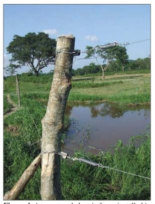
**Figure 4.** A two-strand electric fence installed in Sonitpur district.
